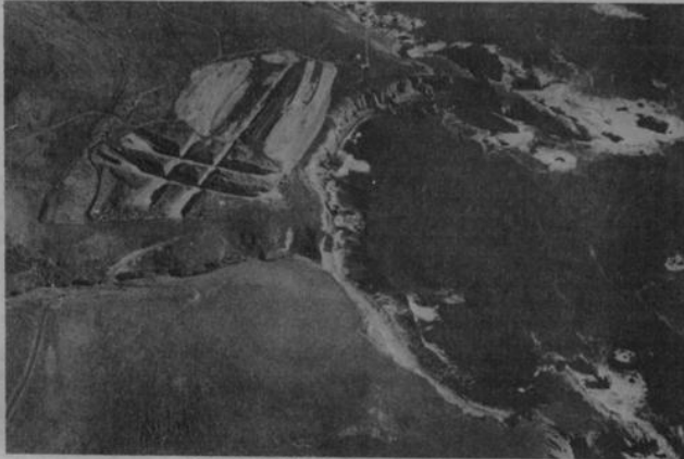
PG&E declined to extend trenches shown in this 1967 photo of Diablo Canyon to trace a fault in cliffs near the mouth of Diablo Creek, to the lower right of the plant site, according to an AEC memo.
