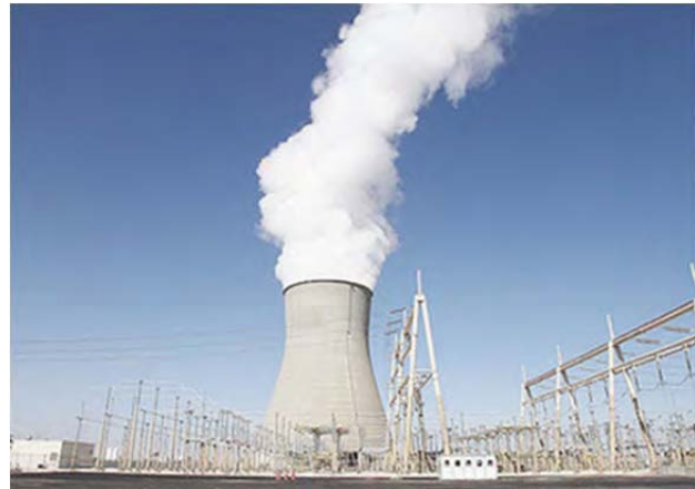
Figure 10. Hope Creek Cooling Tower 56
