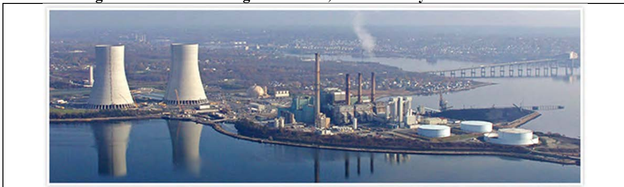
Figure 4. Retrofit cooling towers at 1,500 MW Brayton Point Station 22
