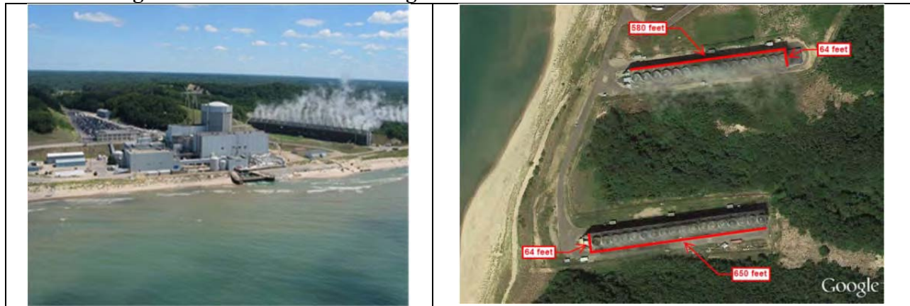
Figure 3. Retrofit inline cooling tower at 800 MW Palisades Nuclear 15,16
