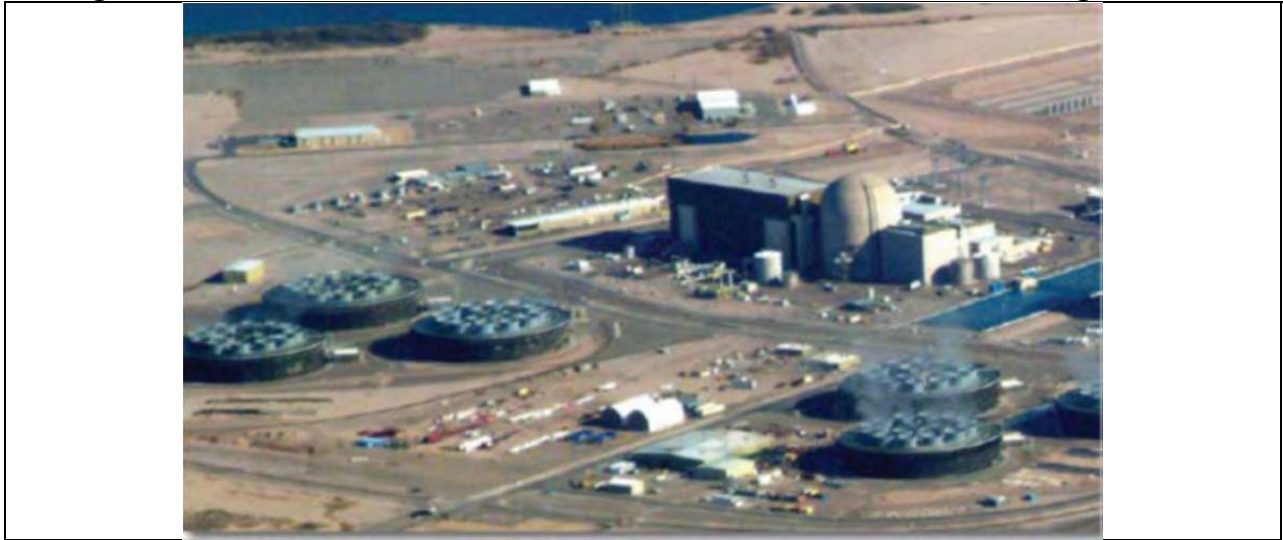
Figure 14. Palo Verde Nuclear Plant with Round Mechanical Draft Cooling Towers 67
