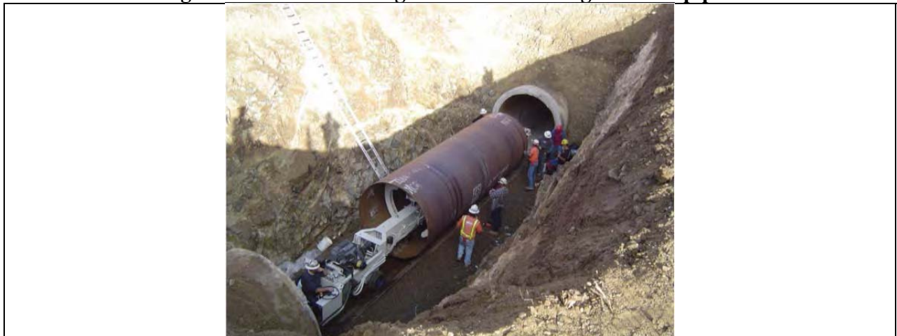
Figure 2. Steel liner being inserted in existing concrete pipe 12
