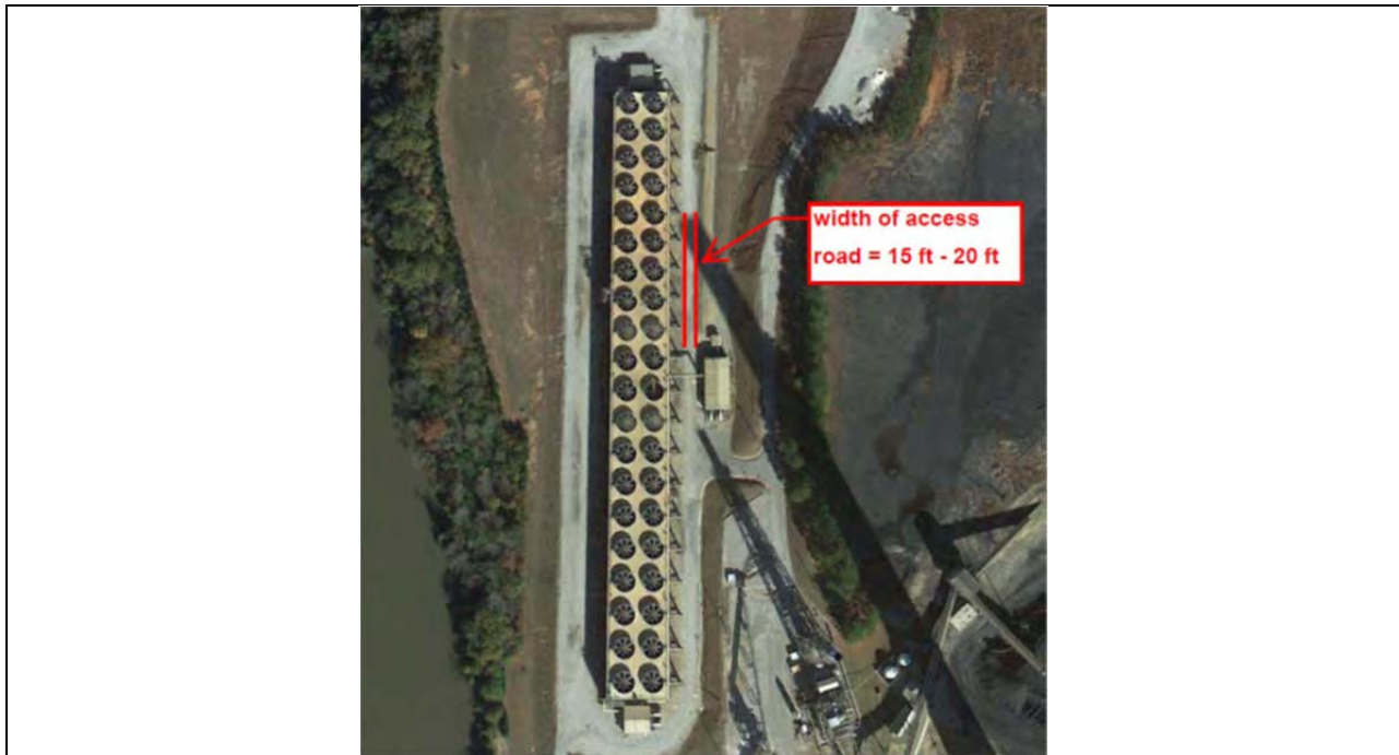
Figure 10. Plant Yates 40-cell back-to-back cooling tower with 15- to 20-foot wide access road on one side 54
